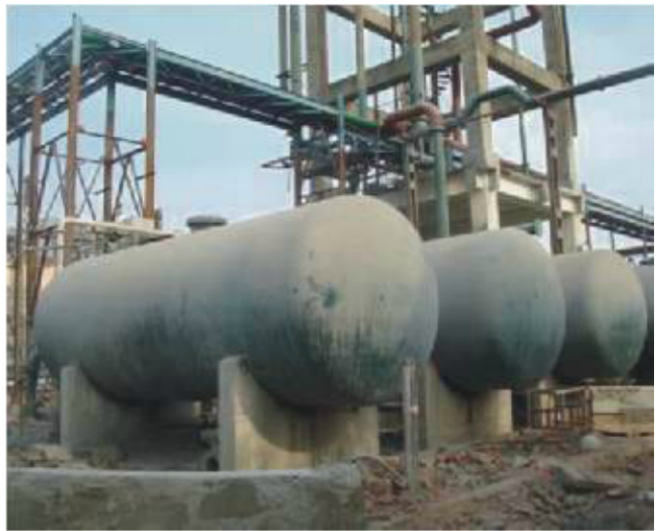
Final Picture of DM Plant After Demolition
