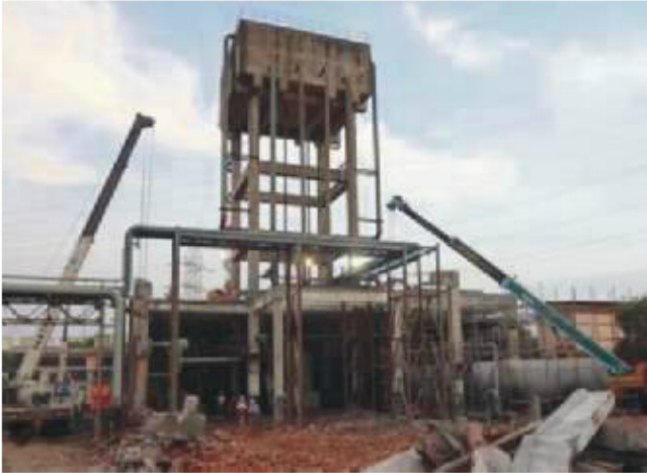
Two Cranes Working in Tandem
