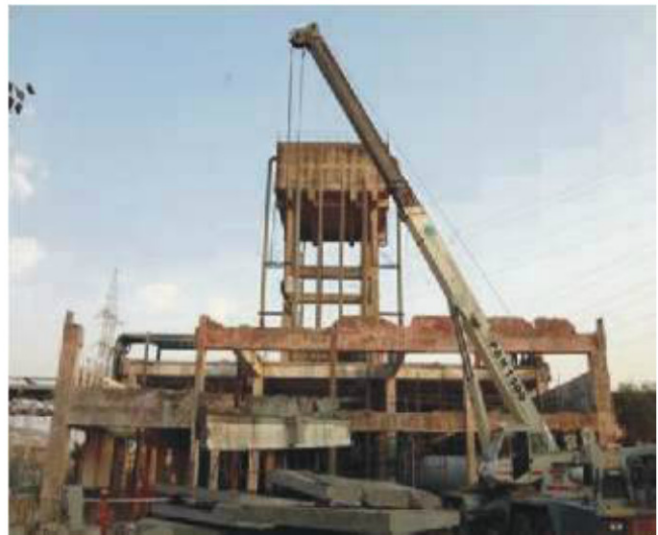
Lifting and Lower of cut pieces after cutting
