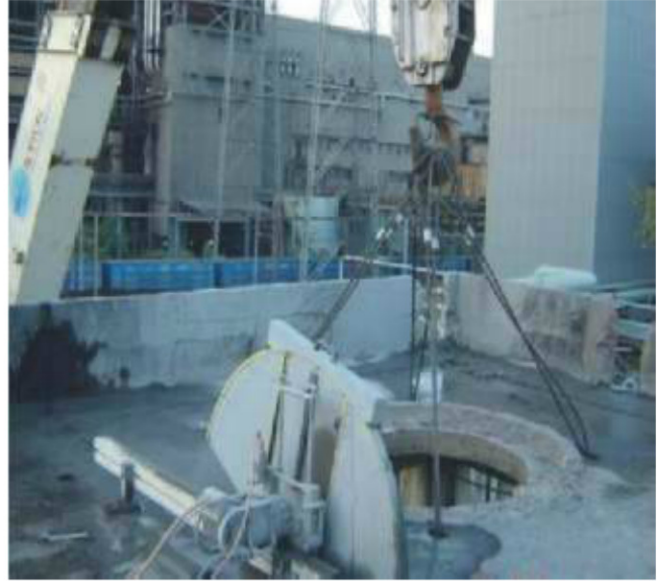
Wall Sawing of RCC Slab
