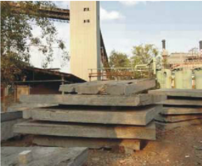
Picture of Slabs After Diamond Cutting
