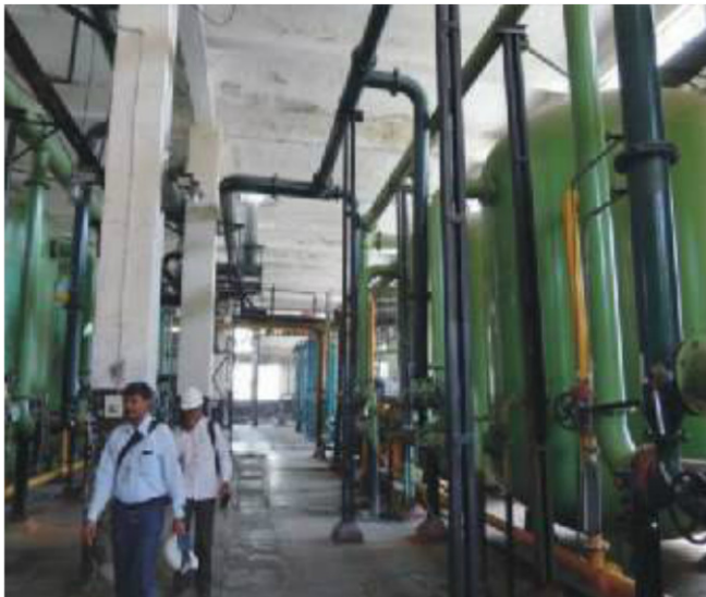
Pictures of DE Mineralization Plant before start of the job showing the Pressure Vessels etc.,
