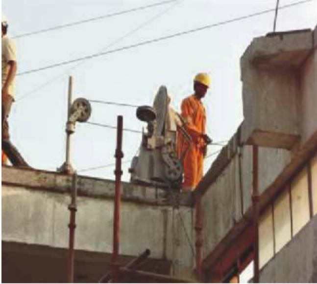
Wire Sawing of Beams
